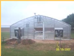
Greenhouse nears completion
